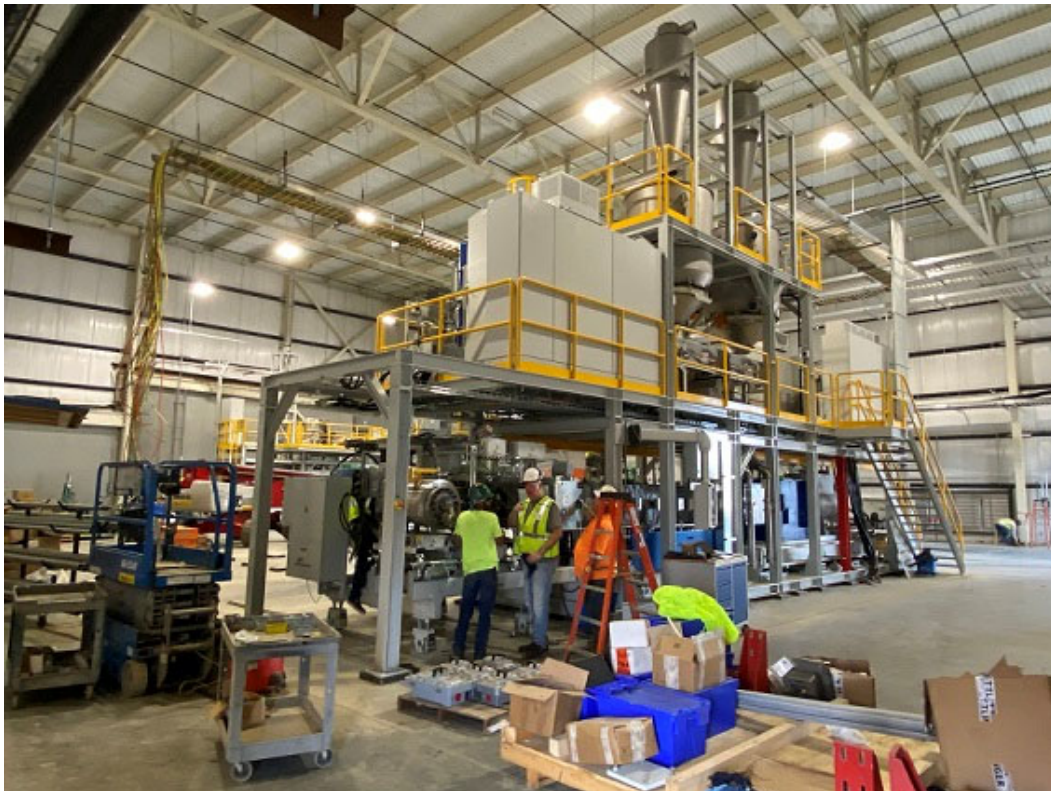
Figure 4: Installation of Extruder in Building 610
