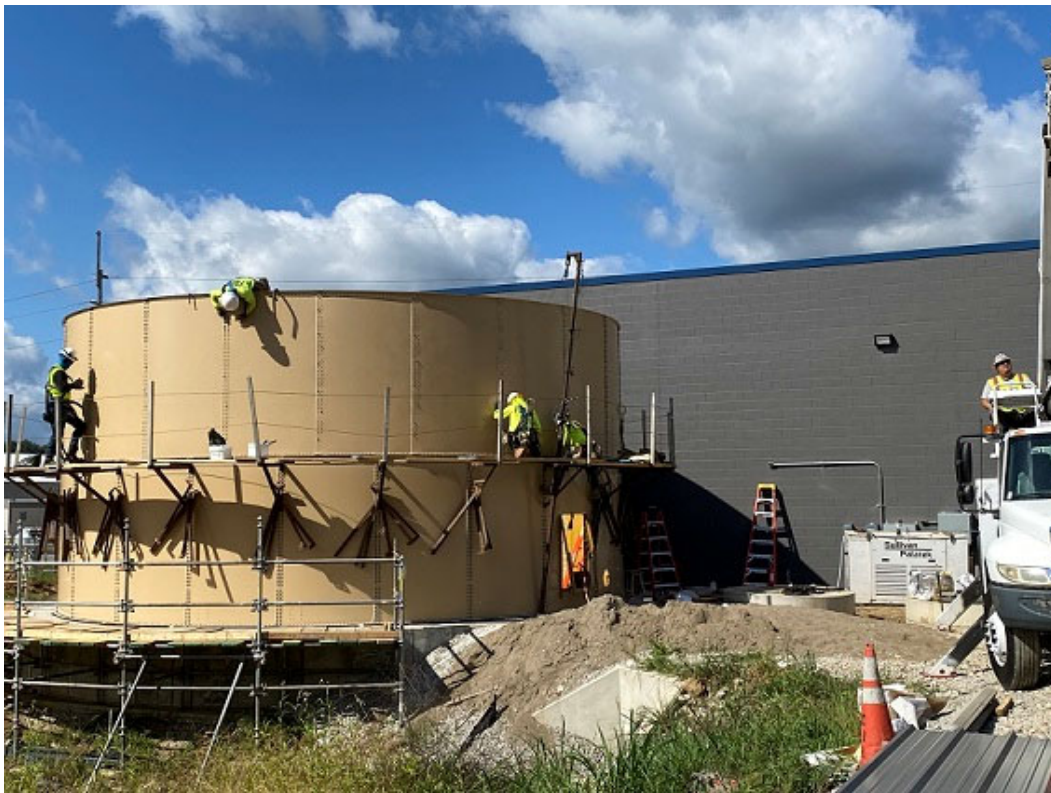
Figure 6: Installation of WWPT Tank
