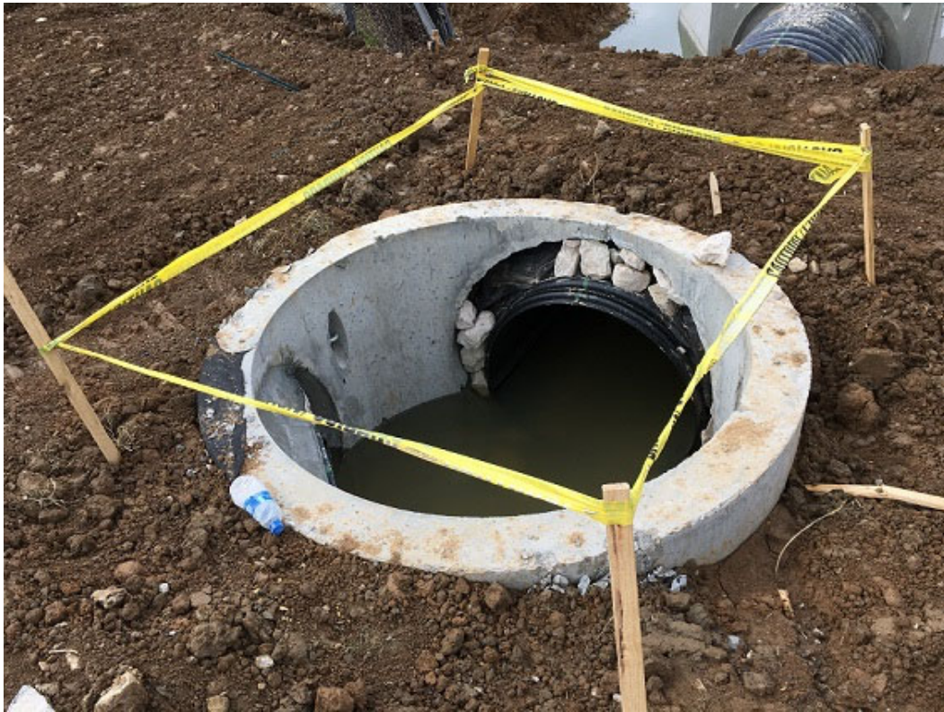
Figure 6: Stormwater Drainage Installation
