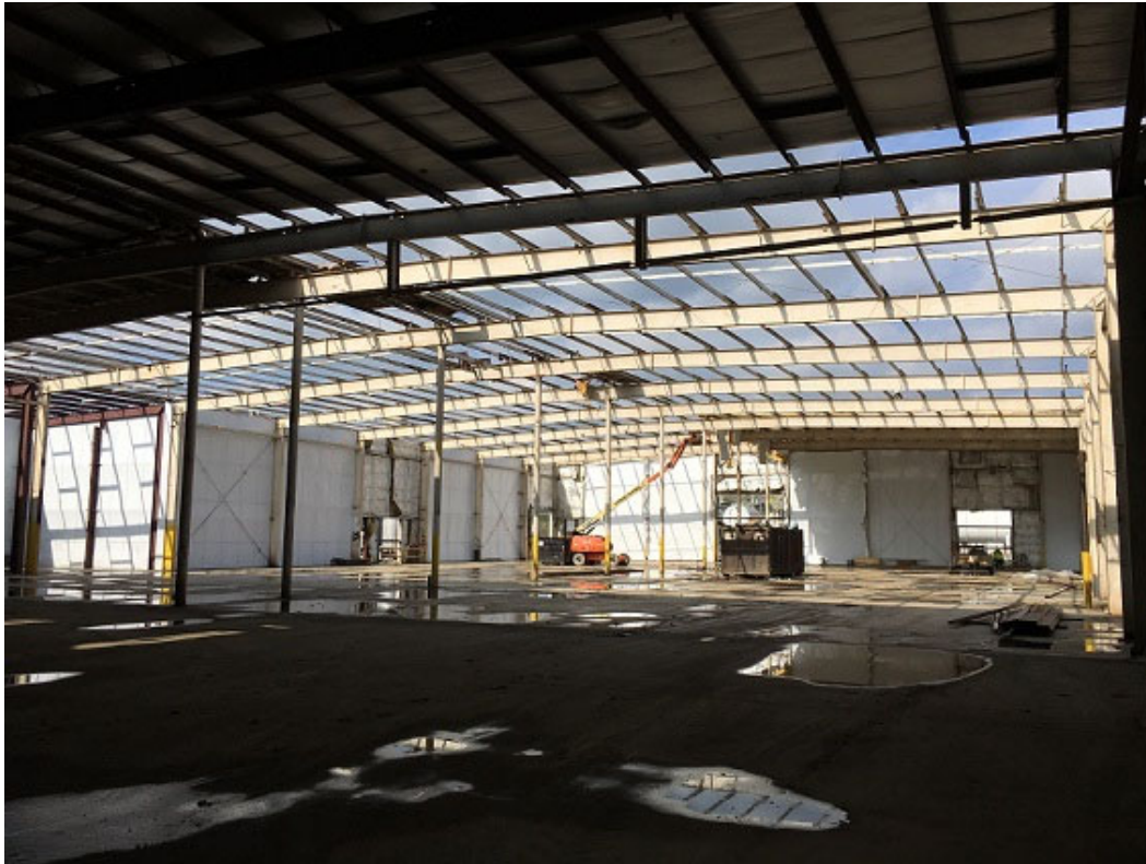
Figure 2: Building 504 Roof Deck Installation
