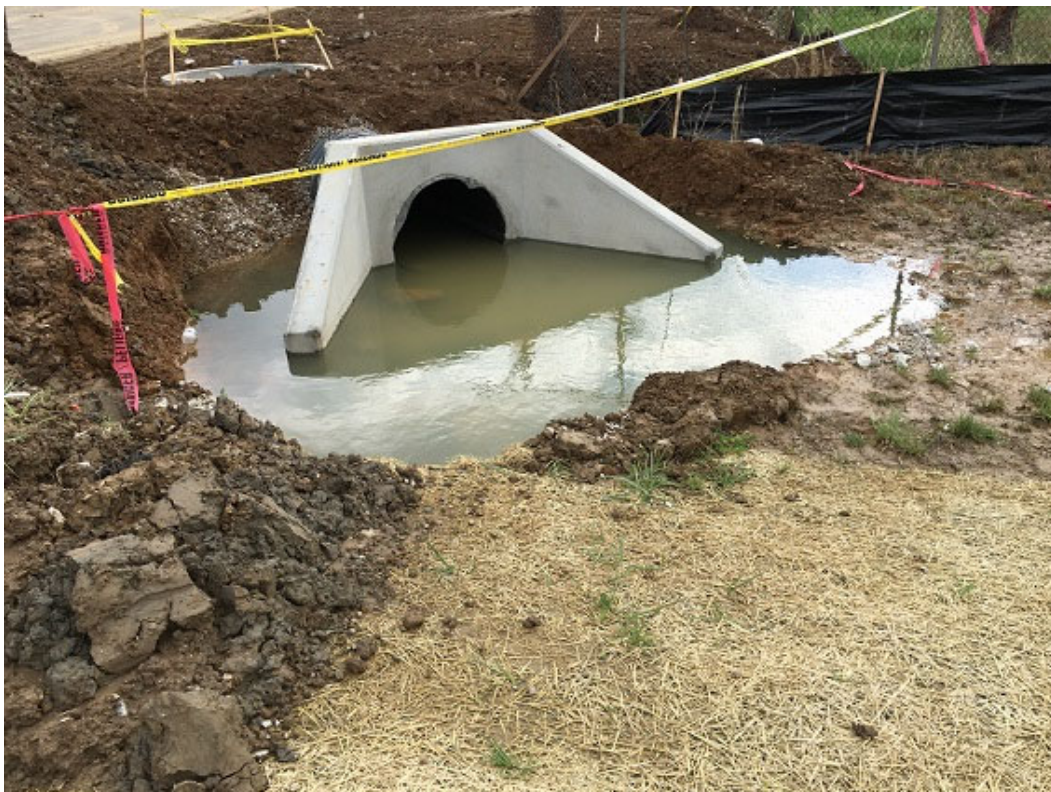
Figure 6: Stormwater Drainage Installation
