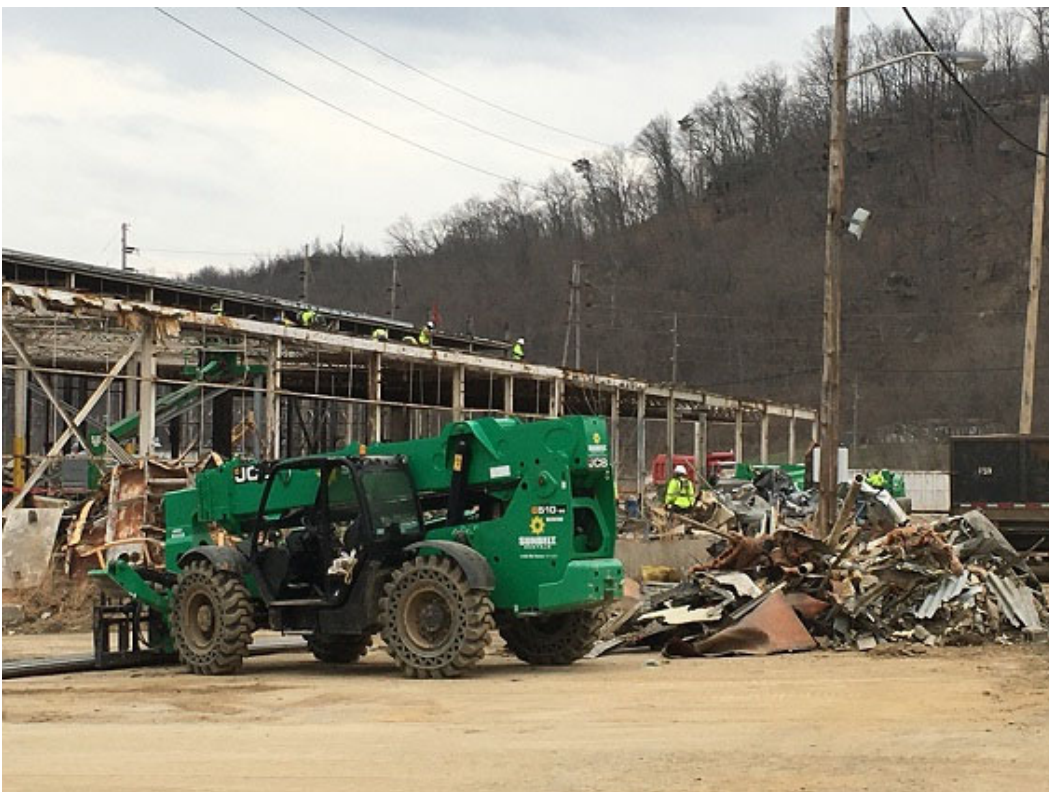
Figure 2: Removal of Demolition Debris
