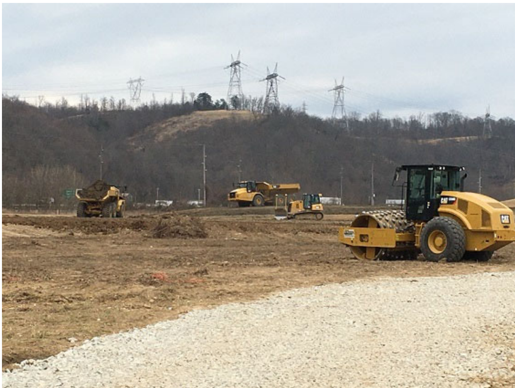
Figure 6: Mass Grading Equipment
