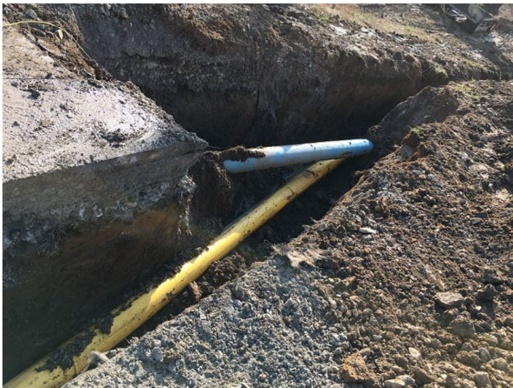
Figure 2: Installation of Fuel Gas Line to Facility
