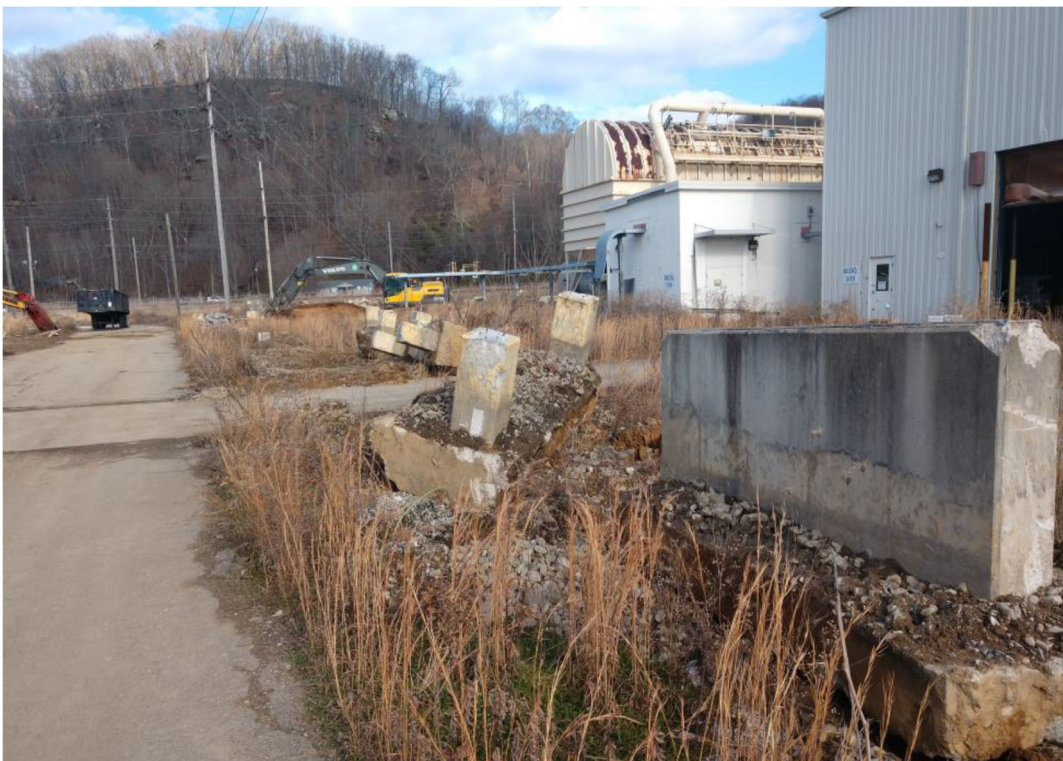
Figure 4: Demolition of Existing Foundations
