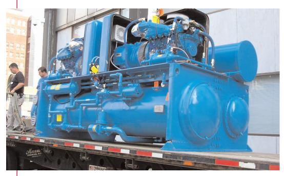
When the time came to replace the building's old chiller plant, the City opted to put in a hybrid natural gas and electric cooling system. Two Tecogen TECOCHILL CH-400x chillers were installed along with a 600-ton electric chiller.
