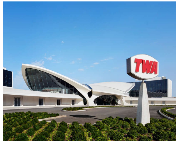
The TWA Hotel overlooks runways at the JFK International Airport and the TWA Flight Center.
