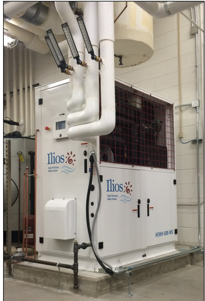
The Ilios HEWH-500-WS has a small 3' x 5' footprint which allows it to be easily retrofit into tight existing mechanical spaces as an energy efficiency measure.
