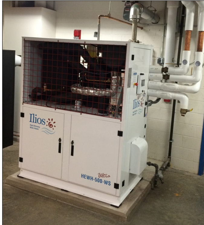
The Ilios HEWH-500-WS's small foot print allows it to be easily retrofit into existing facilities as an energy savings measure.
