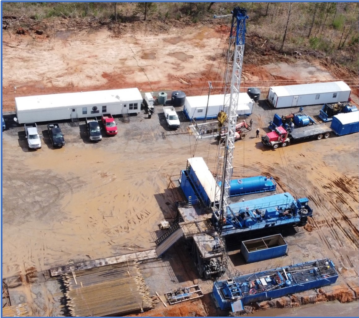
Figure 1: Drill rig at the Beulah-Taylor #1 well re-entry site in Lafayette County, Arkansas. This reused a pre-existing drill pad (note existing powerline running through the wellpad area). The drill rig has since demobilized from this location after reaching a total measured depth of 8,940 ft, and has been replaced by a workover rig to complete perforations, final testwork and sampling.
