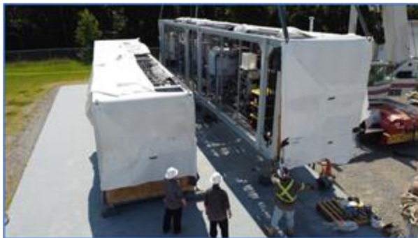
One of the SiFT lithium carbonate crystallization plant modules being lowered into position at Standard Lithium's Demonstration Plant in El Dorado, Arkansas, USA.
