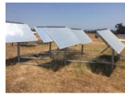
1) Off-the-Shelf Sun-tracking Heliostats (~4 acres per 400 kW)
