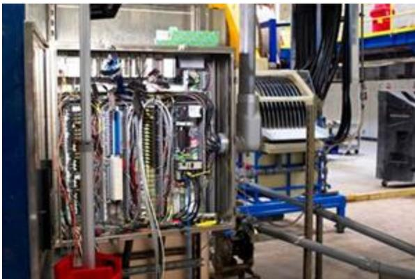
**Pictured is the new AquaRefining automation and control hardware which will reduce the need for manual labor, improving reliability and operating costs.**
