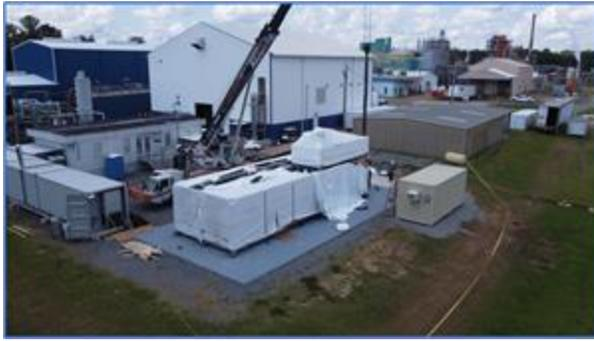
**The final module being loaded into position, with the Company's LiSTR DLE Plant behind. Note the climate-controlled container adjacent to the SIFT Plant, which will be used to store battery-quality lithium carbonate samples produced by the plant.**
