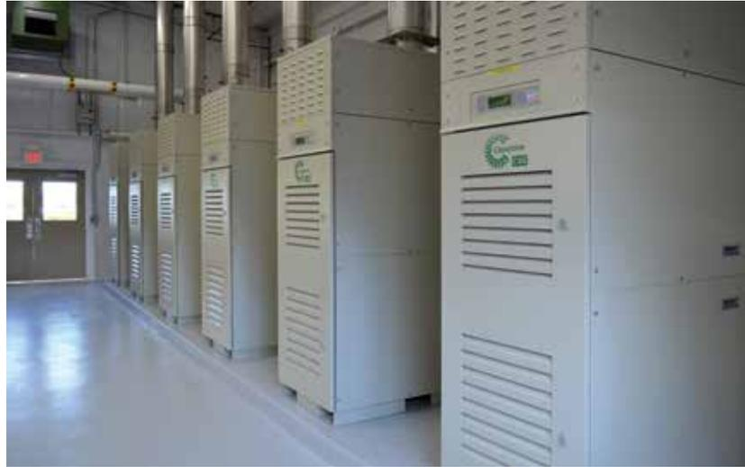
Natural gas fuels six Capstone C65 Integrated CHP microturbines that produce 390kW of clean and reliable power as well as thermal energy for the Viking Yacht Company.
