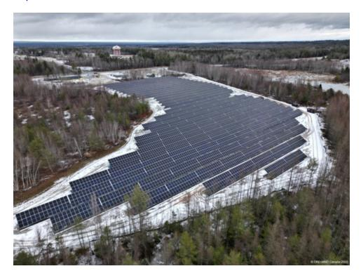
The Gagetown Solar Project, a CAD \$26.7 million initiative. is set to deliver an 8.9 MWdc/7.35 MWac ground-mounted solar energy system designed to provide approximately 8,900 MWh of electricity annually to the base. This project is expected to generate around 20% of the base's electricity needs, significantly contributing to the Department of National Defence's efforts to reduce greenhouse gas
