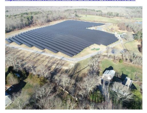
Installed on a former corn field, Ameresco's Tiverton's solar energy site comprises over 12,000 modules with an electricity generation capacity of 4.95 MW.
