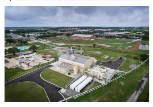
Pictured here, new central plant with microgrid and island mode capability providing 3.5 MW of electric and the full steam load required by MCRD Parris Island. (Photo: Business Wire)
