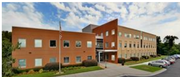
GSA Social Security Administration Building, 5850 Lake Herbert Drive, Norfolk, Virginia
