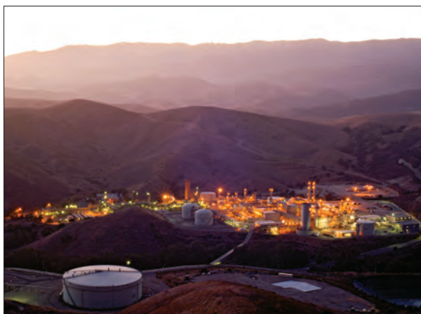
Production from our Santa Ynez Unit offshore development is processed at the Las Flores Canyon Plant in California.
