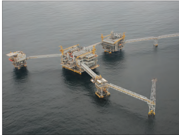
Natural gas liquids are produced from the East Area Complex in Nigeria.
