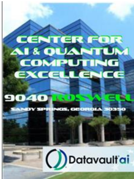
Datavault AI's Center for AI and Quantum Computing Excellence in Sandy Springs, Georgia
