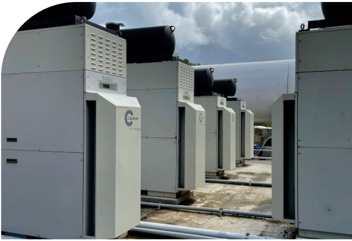
Seven propane-fueled microturbines produce 1-million kWh of electricity annually and over a billion BTUs in hot water for Magens Junction, an affordable housing development in St. Thomas.
