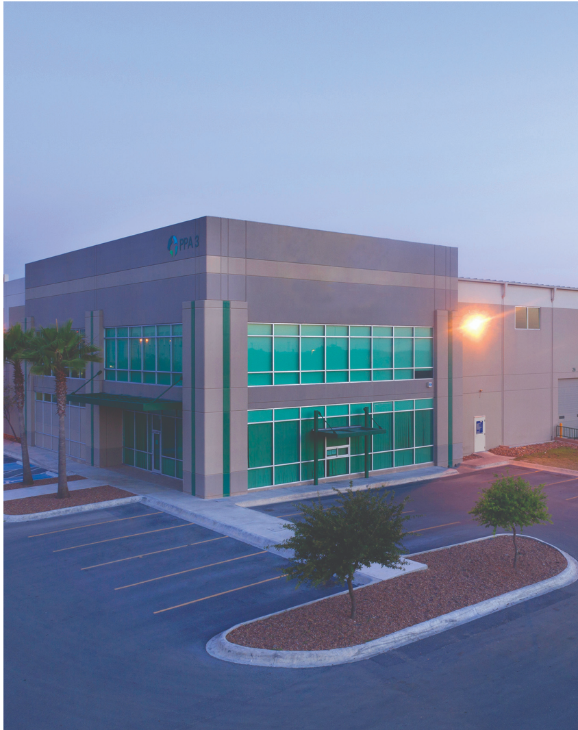
Apodaca Building 3, Monterrey, México
