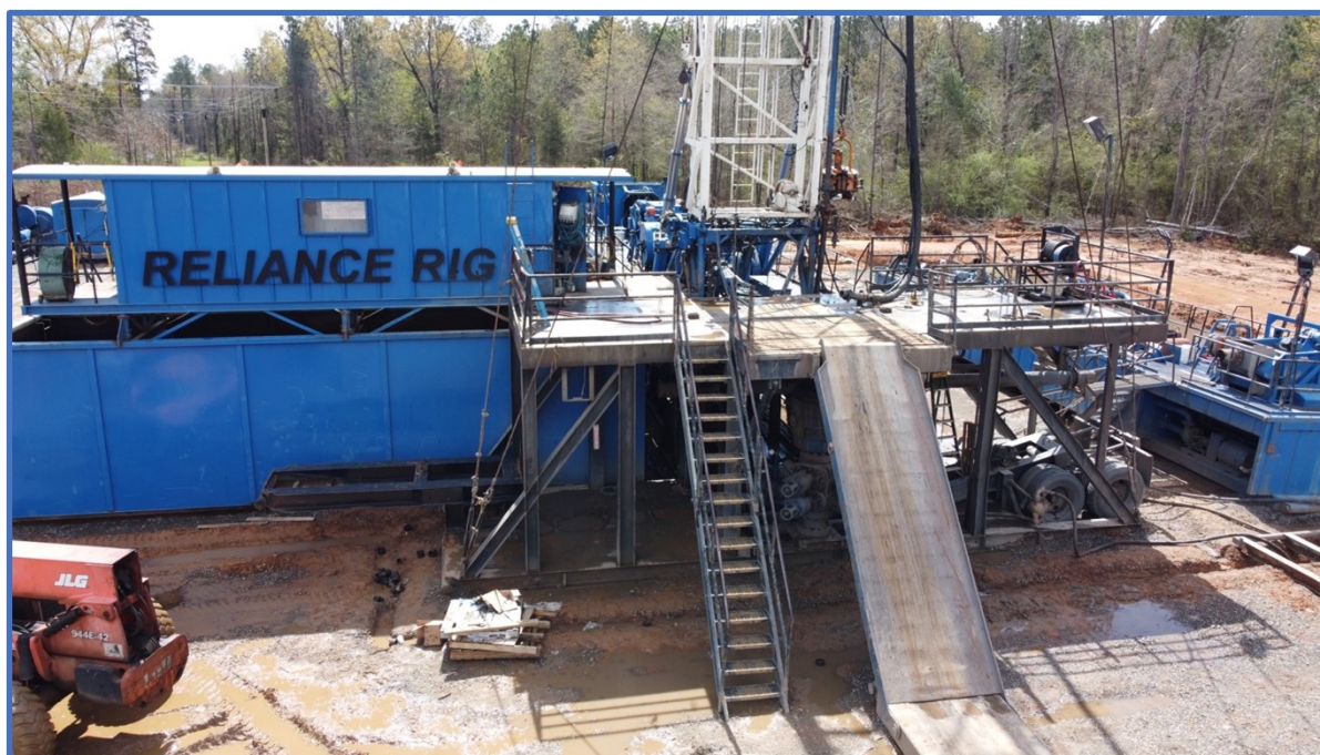
Figure 2: Close-up of the drill rig used to re-enter and deepen the pre-existing Beulah-Taylor #1 well.
