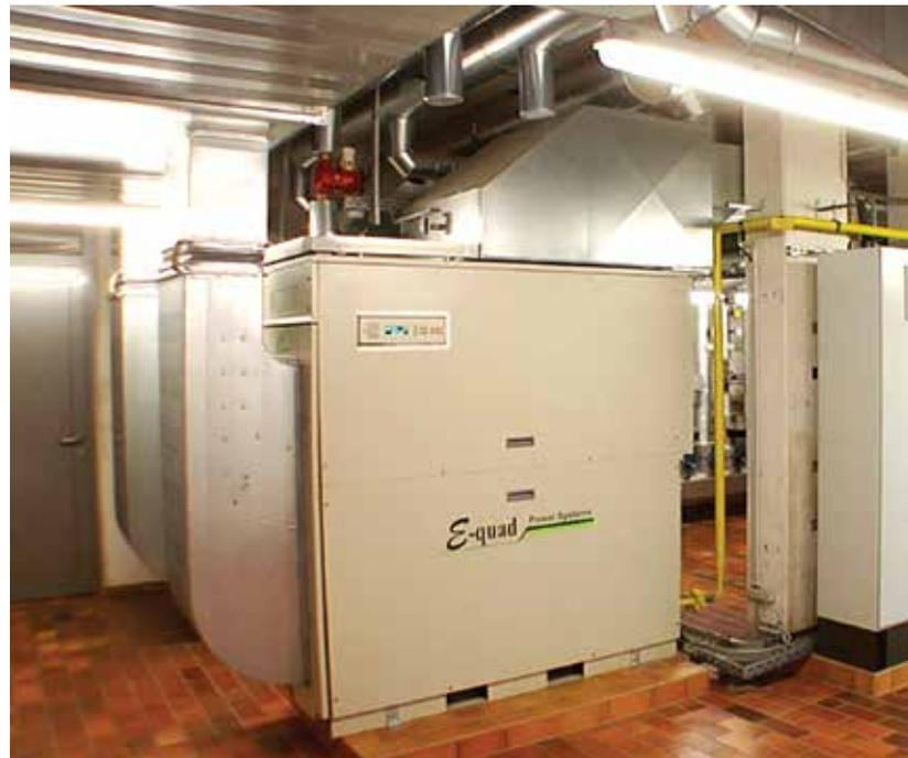
Two natural gas Capstone C65 microturbines make up the combined heat and power system at Catholic Hospital Koblenz in Augsburg, Germany.
