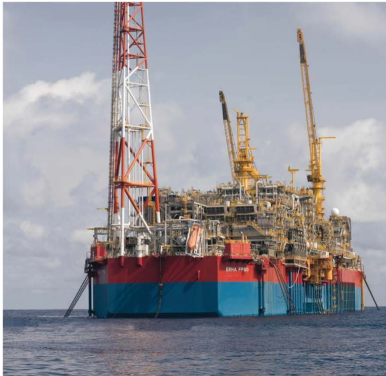
Erha FPSO, offshore Nigeria
