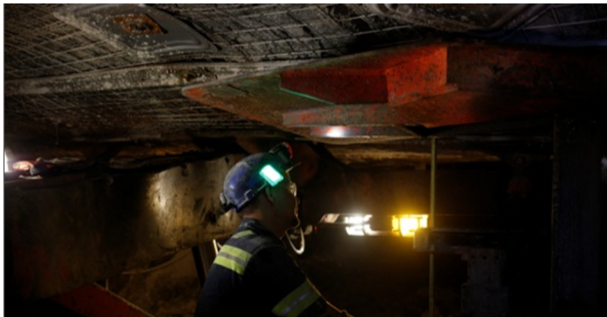
Image 3: Roof bolting operations
