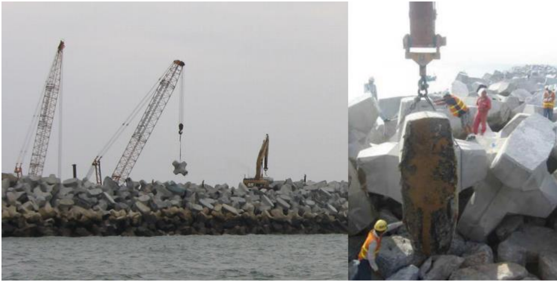
FIGURE 4: CONVENTIONAL ACCROPODE PLACEMENT DUNG QUAT BREAKWATER, VIETNAM
