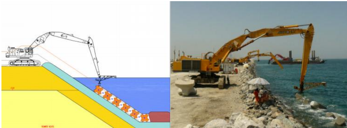
FIGURE 12: PLACEMENT AROUND THE WATERLINE
