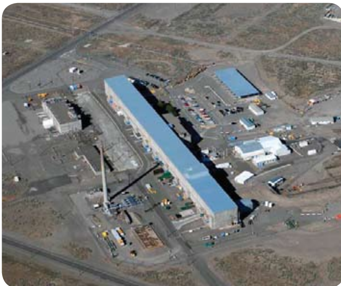
T plant at the Hanford site
