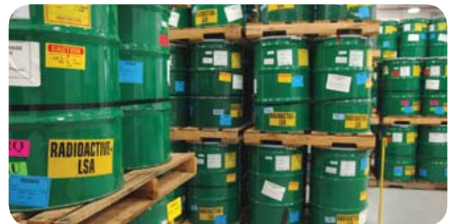
Radioactive drums at our M&EC facility
