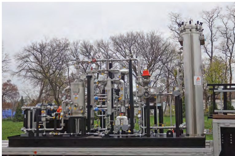
A new Unison gas cleanup skid protects the equipment from siloxanes and condensation.
