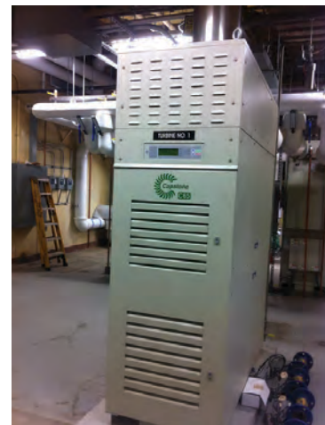
Two 1987-era engines were replaced by four energy-efficient Capstone microturbines.
