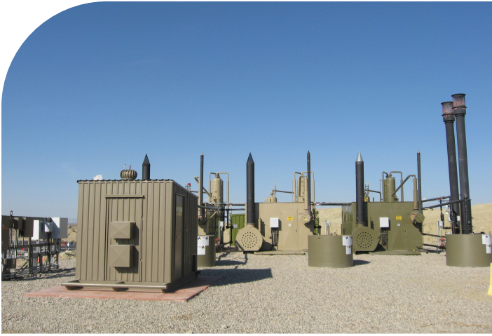
Capstone C30 microturbines at 14 remote Jonah Field well sites generate electricity to power production equipment.
