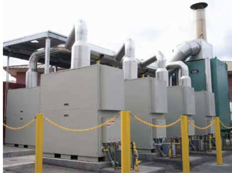
Eight Capstone C60 microturbines provide combined cooling, heating and power to EMWD's Operations and Maintenance Center in Perris, California, while a ninth microturbine provides combined heat and power to the facility.
