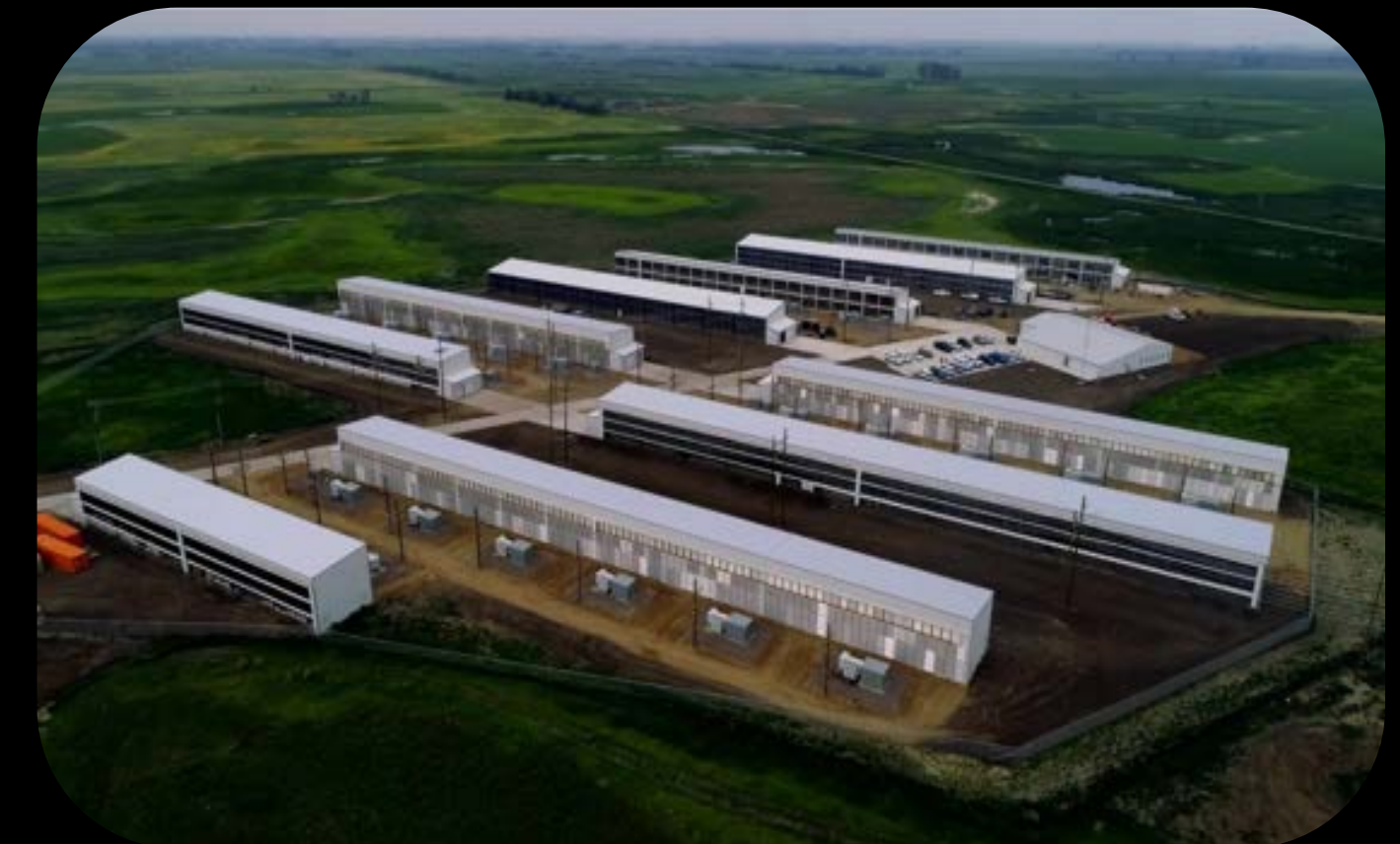
Ellendale, North Dakota Facility 180MWs
