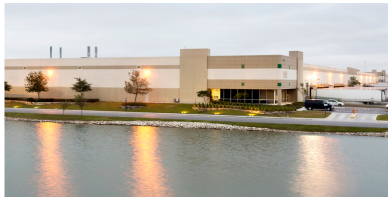
Prologis Pharr Bridge, Reynosa, Tamaulipas.
