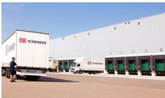
Prologis Park Ausgurg, Munich, Germany
