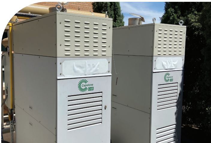
Two C65 microturbines fueled by low-pressure natural gas provides Salt Lake Community College, located in Utah, reliable power while also reducing energy cost.
