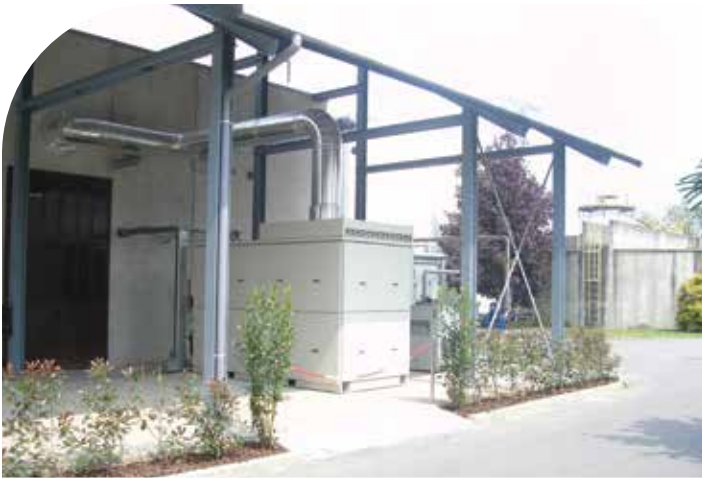
A single Capstone CR200 microturbine fueled by biogas provides all the electrical power needed at the Cossato Spolina Wastewater plant in Italy.
