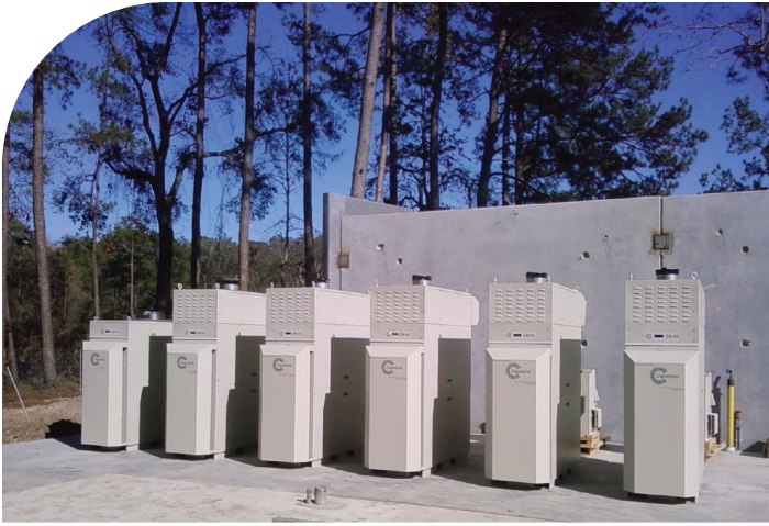
Six Capstone C65 microturbines generate continuous power at this U.S. government office.
