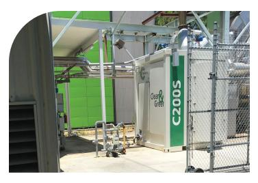
A C200S microturbine is operated in a CCHP configuration, generating onsite electricity and recovering waste heat to power two 30-RT, hot-waterfired absorption chillers that base load the plant's heating, ventilation and air conditioning system.
