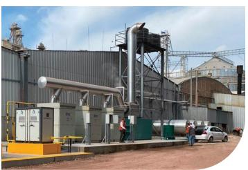
and produces hot air at 280°C (536°F) with an energy of 2.97 GJ / hour. The hot air is then channeled to a Cain Industries steam generator that serves as an auxiliary to two existing boilers in the Forrajera, used in the heating and cooking of its feed production.
