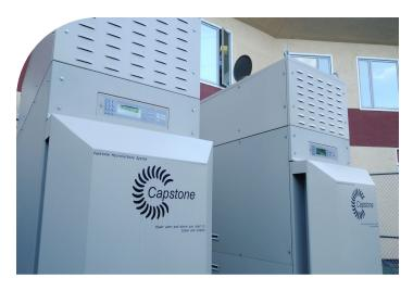
Two C65 ICHP microturbines provide all of the medical facility's thermal and electrical needs, decreasing their carbon footprint by more than 70% and reducing noise pollution.
