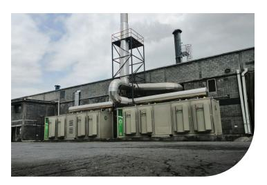
the microturbine's exhaust gases for use in the egg carton drying ovens—an added operational efficiency that resulted in greater than expected savings in a short amount of time.
