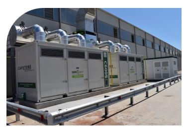
The electricity generated by two C600S microturbines meets the base demand of the manufacturing plant, while the exhaust gases are fed into a brick dryer, providing heat for the manufacturing process.
