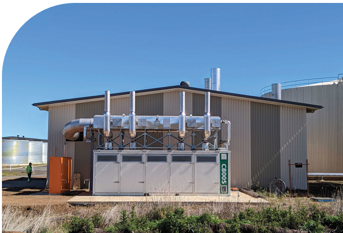
The Capstone C800S microturbine system at Costa Group's facility provides 800kW of reliable power while operating as a highly efficient CHP (combined heat and power) and CO2 fertigation solution.
