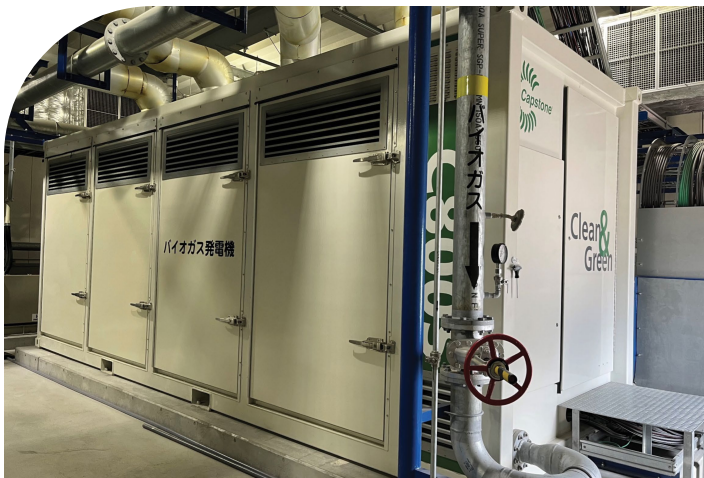
The C800S Signature Series microturbine at Biokurasix Handa converts agricultural waste into clean power, heat, and CO 2 for sustainable farming, showcasing a high-efficiency biogas energy model in Japan.
