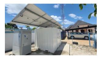
Modular, compact, very expandable, presently configured for 70 kW peak power and 18 kW continuous power
