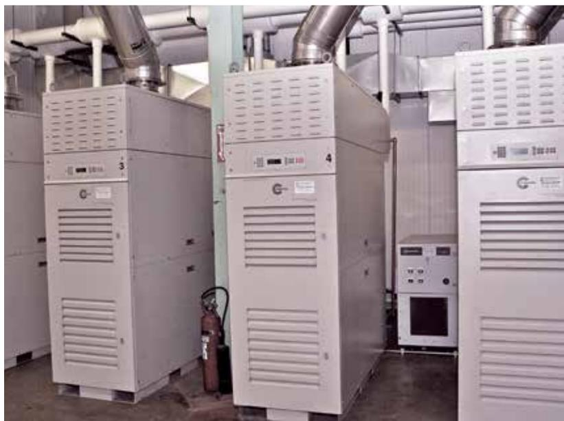
*Capstone microturbines provide cooling, heating, and power at Astor Chocolate in New Jersey.*
