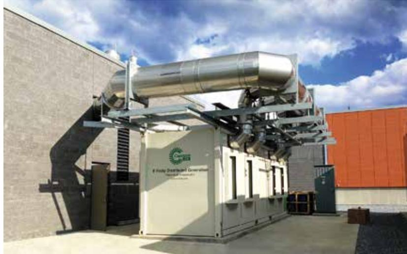
A Capstone C800 microturbine operating in a CCHP application producing 800kW of clean and reliable power for the PSECU data center UPS.
