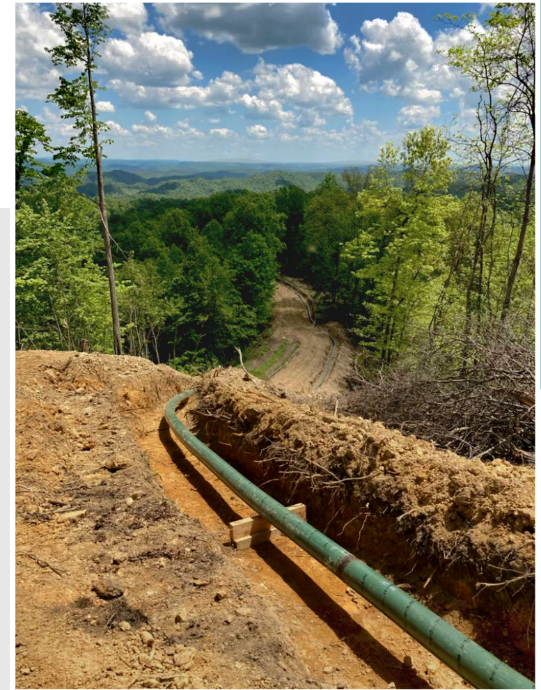
Company Image: Installation of new transportation pipeline
