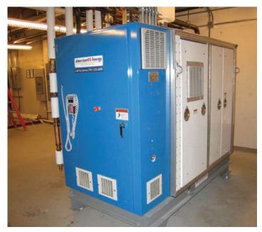
The CHP on-site utility model provides a system at no cost to the customer. The supplier takes full responsibility for operating and maintaining the system. (This CHP unit was recently installed at the Hotel Indigo in Newton, Mass.)
