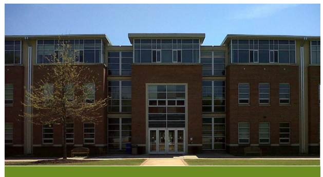
Cleanliness is a priority of Woodward Academy in Atlanta, which specified antimicrobial-coated steel for its rectangular ductwork to inhibit the growth of microbes.
